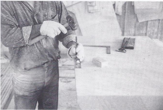
3 Square up the chipped area into a regular slot.
